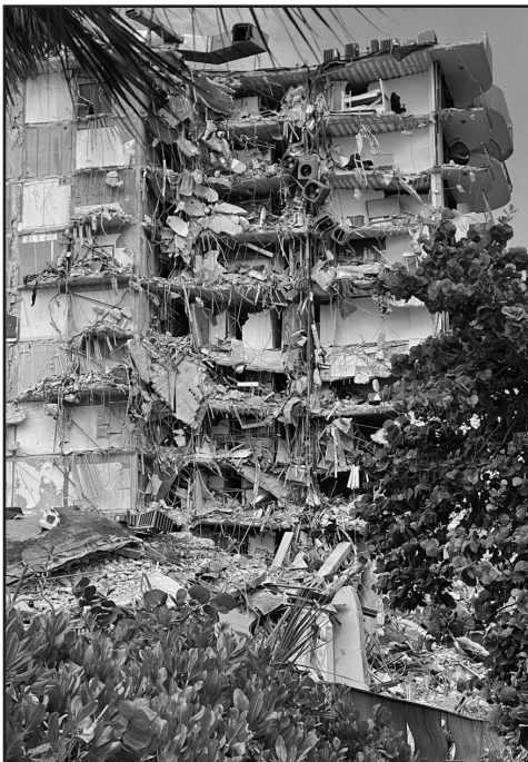
The collapsed Champlain Tower South, Surfside, Florida.
