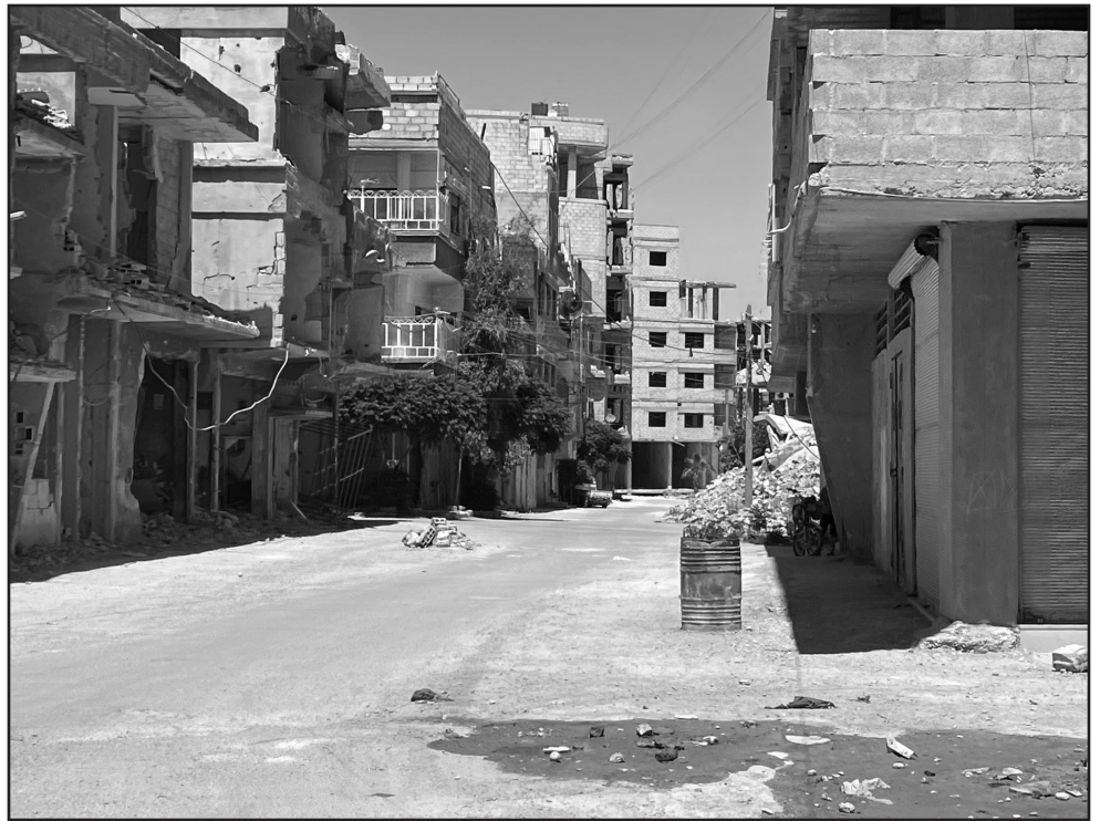
In the badly damaged Jobar neighborhood of Damascus, restorations like the charming balconies on a building (third from left) are an inspiring sign of Syrian resilience. Photo: Wyatt Miller
